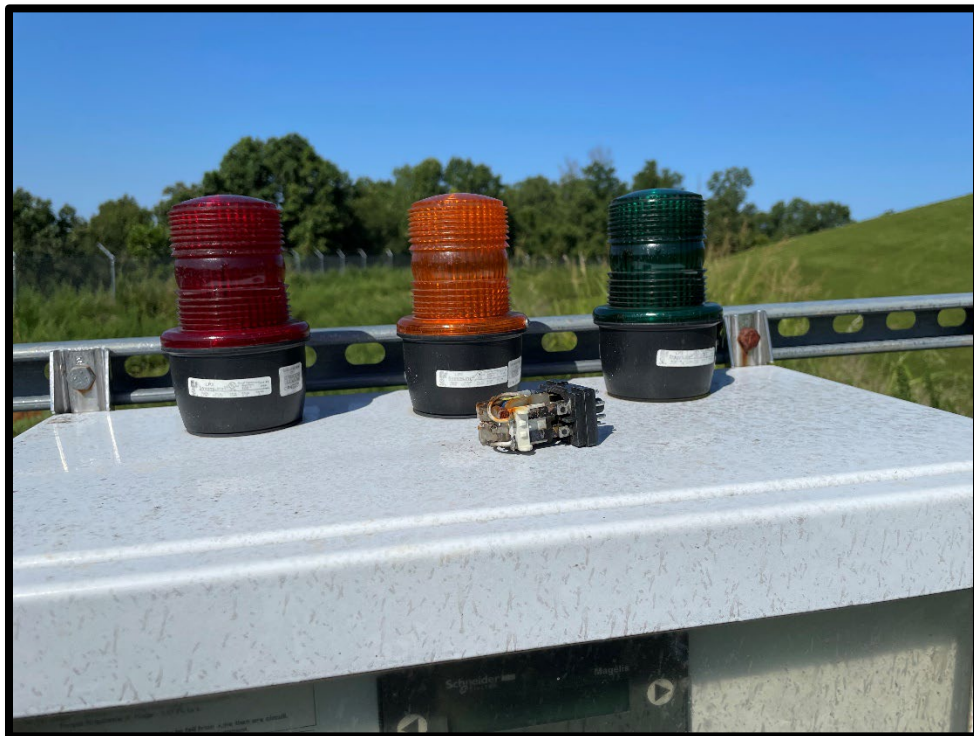
Photograph 8: Damaged electrical part on LCS-2 housing.
