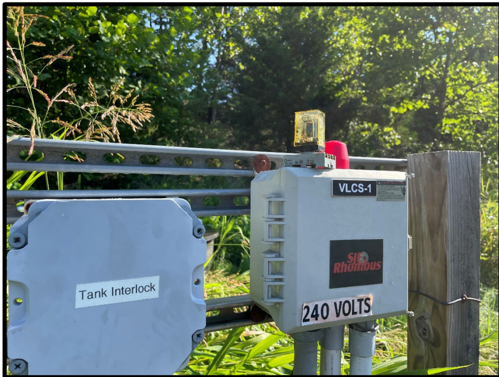
Photograph 6: Damaged electrical part on top of VLCS-1 housing.
